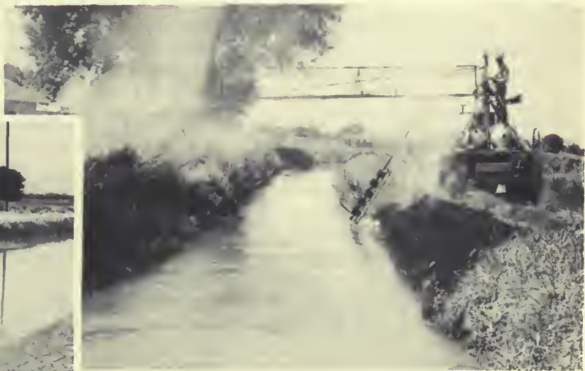
BUTANE-PROPANE burner clearing grass and weeds from lateral banks (at right). Below: Spraying weeds with fortified oil on Franklin Canal, Rio Grande project. Both photos by J. G. Koogler, Region 5.
